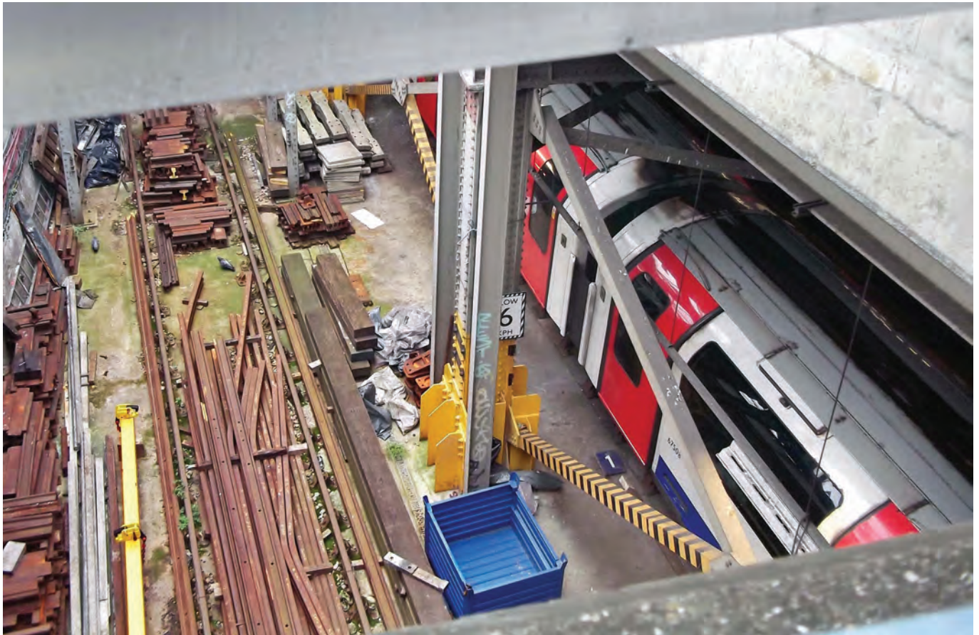
Waterloo and City line access point and sidings at Waterloo station
